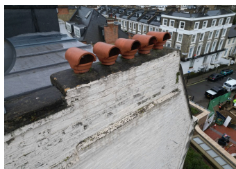
Detail · party wall, pots and weathered capping
