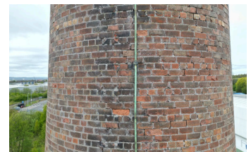
Shaft · pointing, brickwork and conductor tape
